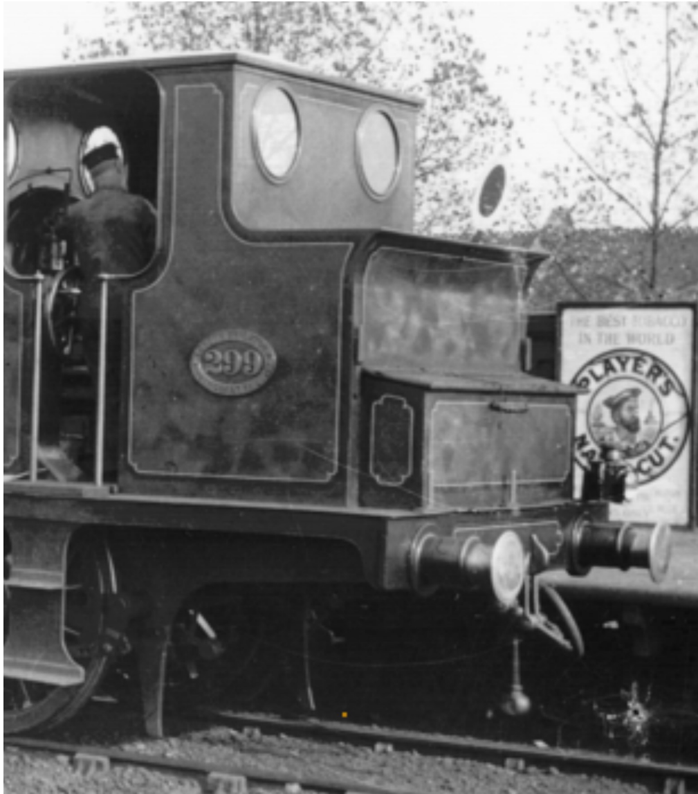
Rear of Stroudley D1, showing additional irons above the tool box.
