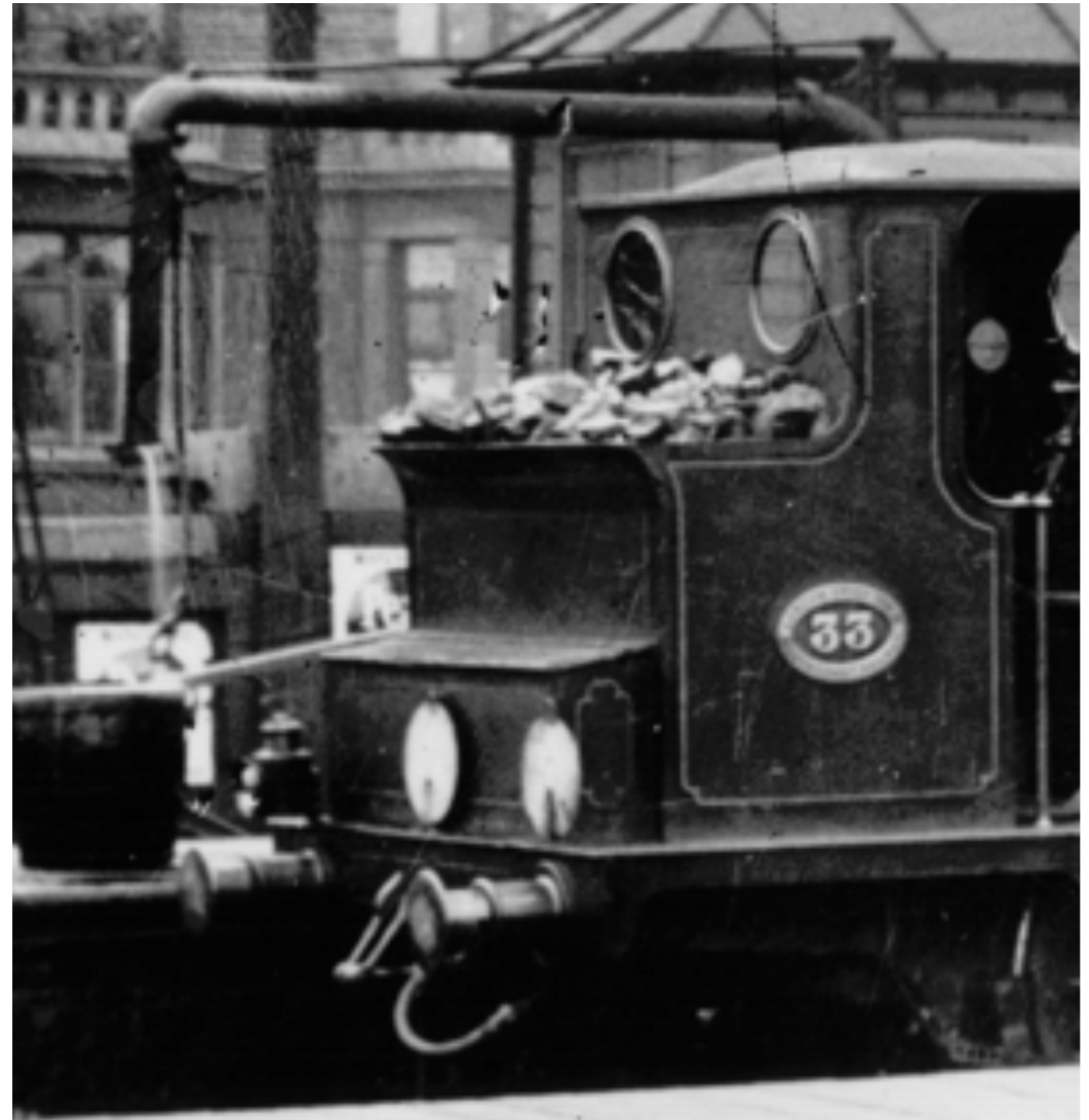
Rear of Stroudley D1, showing all lower lampirons at bufferbeam level and the upper iron on top of the bunker rim.
