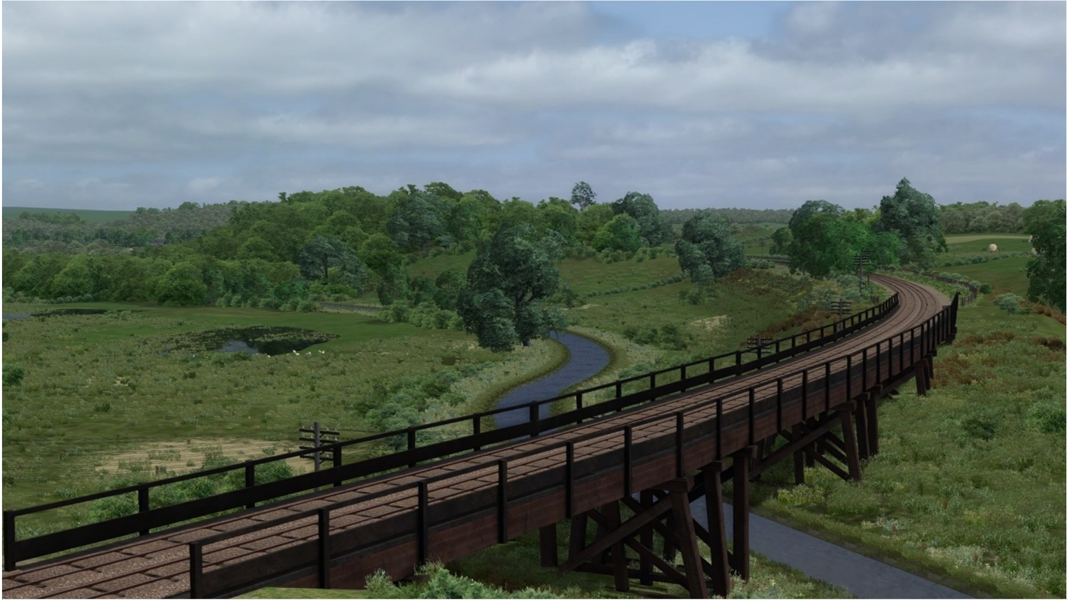
The timber trestle Aedern Valley viaduct
